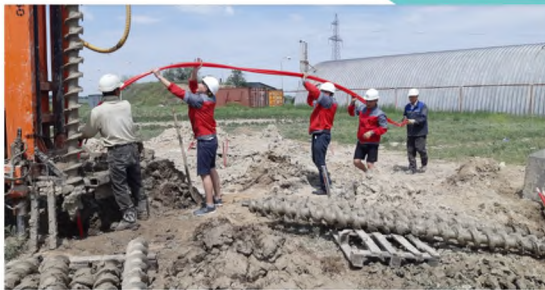
Figure 2. Construction of a ground heat accumulator
